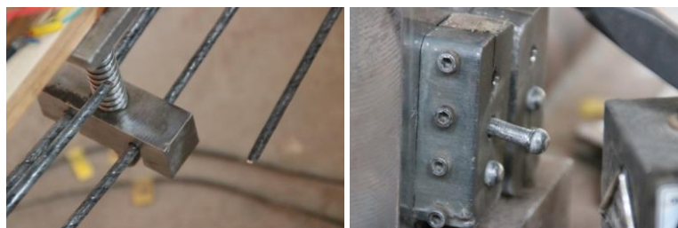
Fig. 2 - The tensile failure of pre-stressing tendons ( L 3-2-3 )
