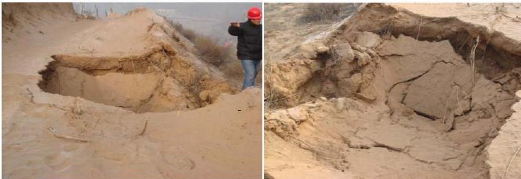
Fig.7 - Surface sandy land in tunnel exit section
