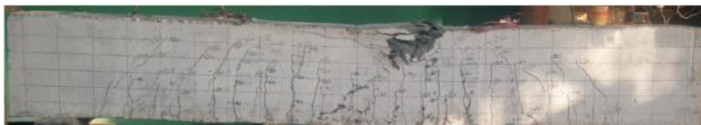
(b) B7 concrete crush
