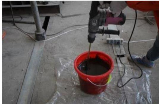
Fig. 1 - Polyurethane cement (PUC) mixing diagram
