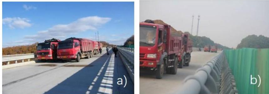
Fig. 6 – Illustration of a) eccentric static loading tests performed before rehabilitation, and b) centric static loading tests performed (b) after rehabilitation
