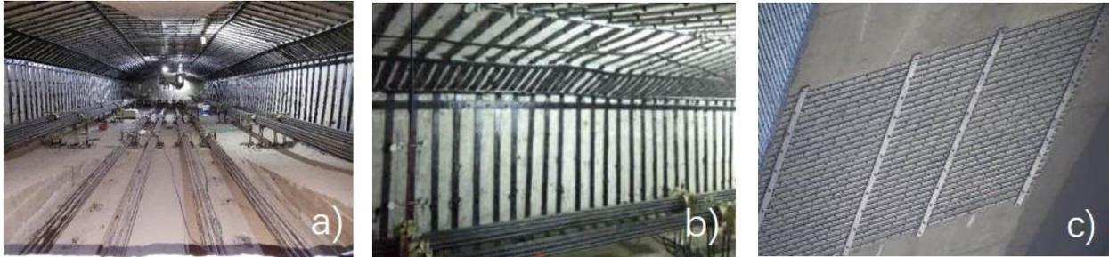
*Fig. 2 – Strengthening of the highway bridge: a) external prestressing, b) steel plates inside the girder, c) steel plates outside the girder.*
